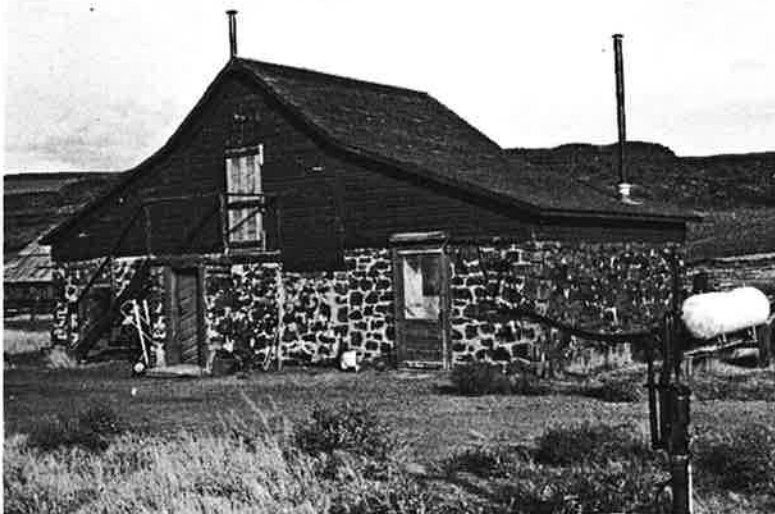
Residence (former bunkhouse and cooler), northeast view: ca. 1907; 43'3"x19'14"; rectangular, one and one-half story, wood frame and masonry structure, uncoursed rubble to second story floor line, wood frame above sheathed with wide shiplap, corner and rake boards. Wood shingle medium gable roof with broad slopes. Narrow one-over-one double-hung sash window, two small rectangular windows on east elevation. Three door openings on west elevation: paneled wooden door offset center to south; one story, central projecting entry, diagonal plank door; stairway to roof of first floor entry provides access to second floor, vertical plank door. No apparent material or structural alterations. Masonry cracked; mortar deteriorating. Fair condition.
