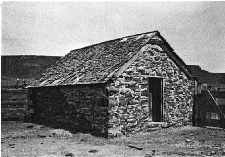
Chicken House, southeast view: ca. 1907; 18'x16'; rectangular, one story stone structure, uncoursed rubble walls 3' thick. Medium gable roof covered with wood shingles. Central, vertical plank door in west gable end. Small, six-light window in south elevation. Roof shingles deteriorating, some missing. Fair condition.
