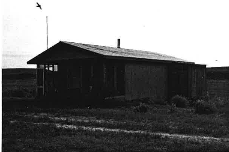
Bunkhouse, west view: ca. 1927; rectangular, one-story, stone foundation, wood frame, sheet metal siding. Vertical wood plank addition on northwest corner, paneled wooden door. Six-over-six double-hung sash window south elevation. Low pitch gable roof covered with sheet metal. Recessed porch on east (gable end) elevation, enclosed with screen, vertical panel door offset center with ornate knob, narrow double-hung sash window with leaded glass. Bird and rodent infestation. Stairway to entrance on west elevation deteriorating. Fair condition.
