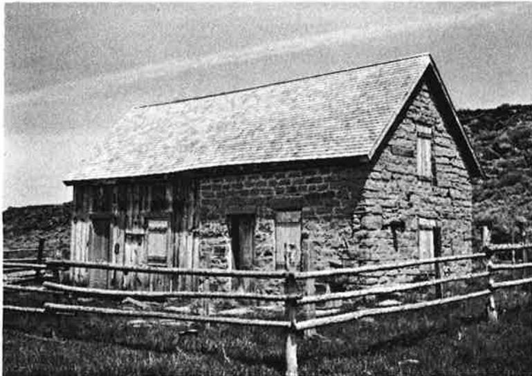
House, northeast view: 34'7" x 16'5"; built in two phases, wood portion to north, constructed ca. 1885, vertical plank walls, most batts missing Southern half, built ca. 1910, coursed, square rubble. Two halves share wood shingle, medium gable roof. Each half has door on west elevation, single leaf, four panel. Window openings boarded up, originally six-over-six double-hung sash on south elevation, openings on other elevations shorter and squattier. Shed roof porch on facade removed, n.d. Severe bird and rodent infestation. Mortar deteriorated, stone wall, south elevation, cracking. Some repair and replacement of materials, not incompatible. Roof resingled 1981. Fair condition.
