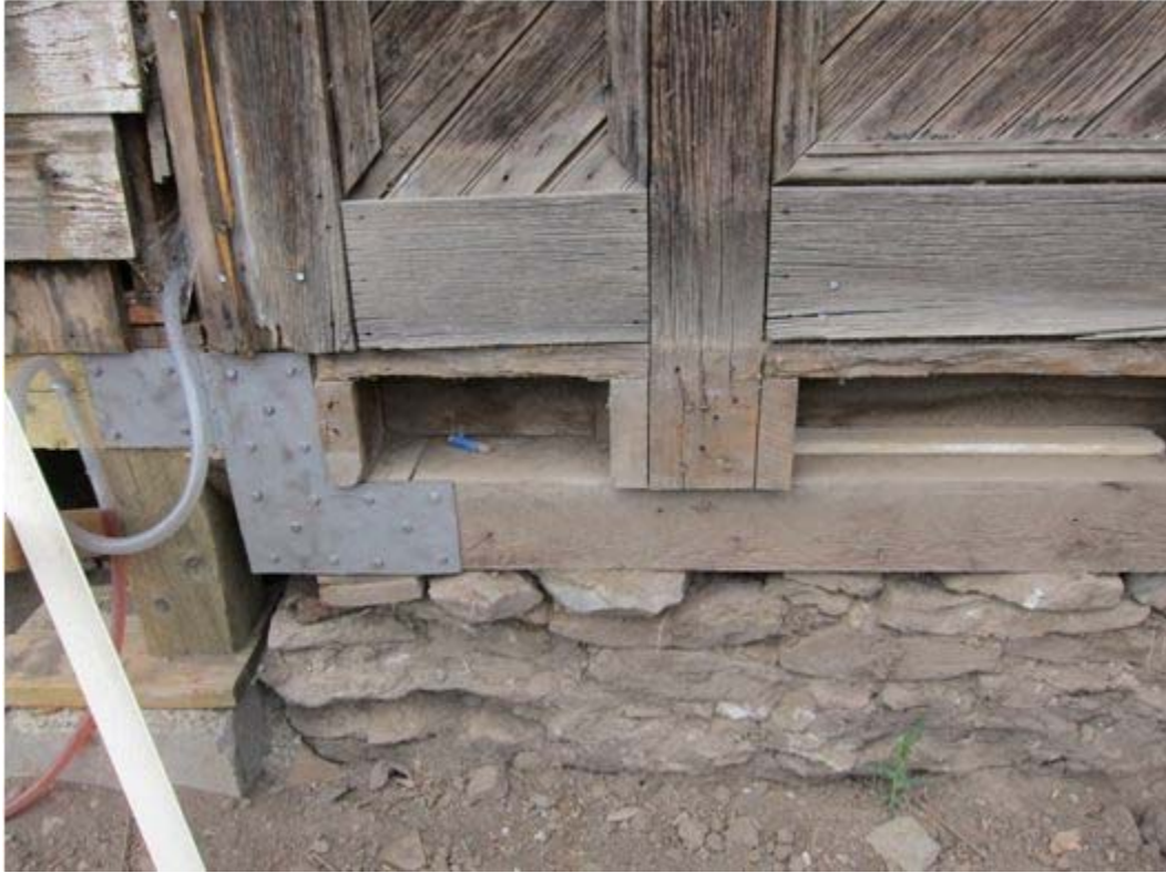
Photo 3 of 16: (OR_MorrowCounty_HardmanIOOLodge_0003) East façade showing close up of rubble foundation and lower storefront windows detailing.
