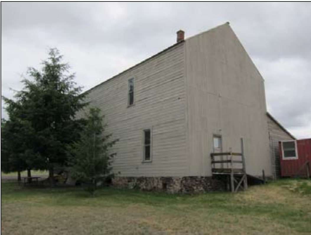
Photo 6 of 16: (OR_MorrowCounty_HardmanIOOFLodge_0006) Looking east at the north and west sides of the lodge.
