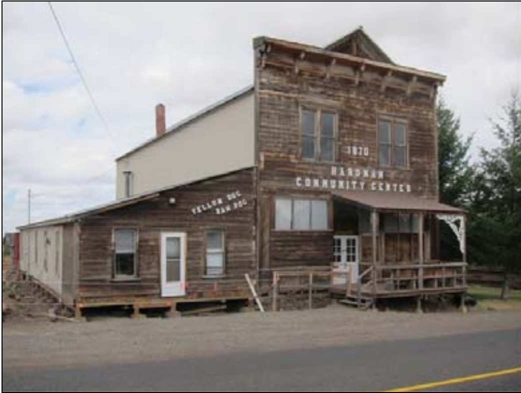
Photo 1 of 16: (OR_MorrowCounty_HardmanIOOFLodge_0001) Looking northwest at the east façade (front) of the Hardman IOOF Lodge Building.
