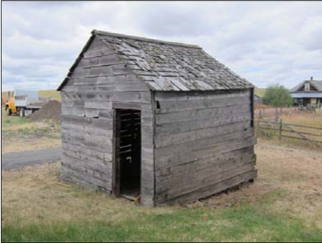
Photo 9 of 16: (OR_MorrowCounty_HardmanIOOFLodge_0009) Looking northwest at the woodshed behind the lodge building.
