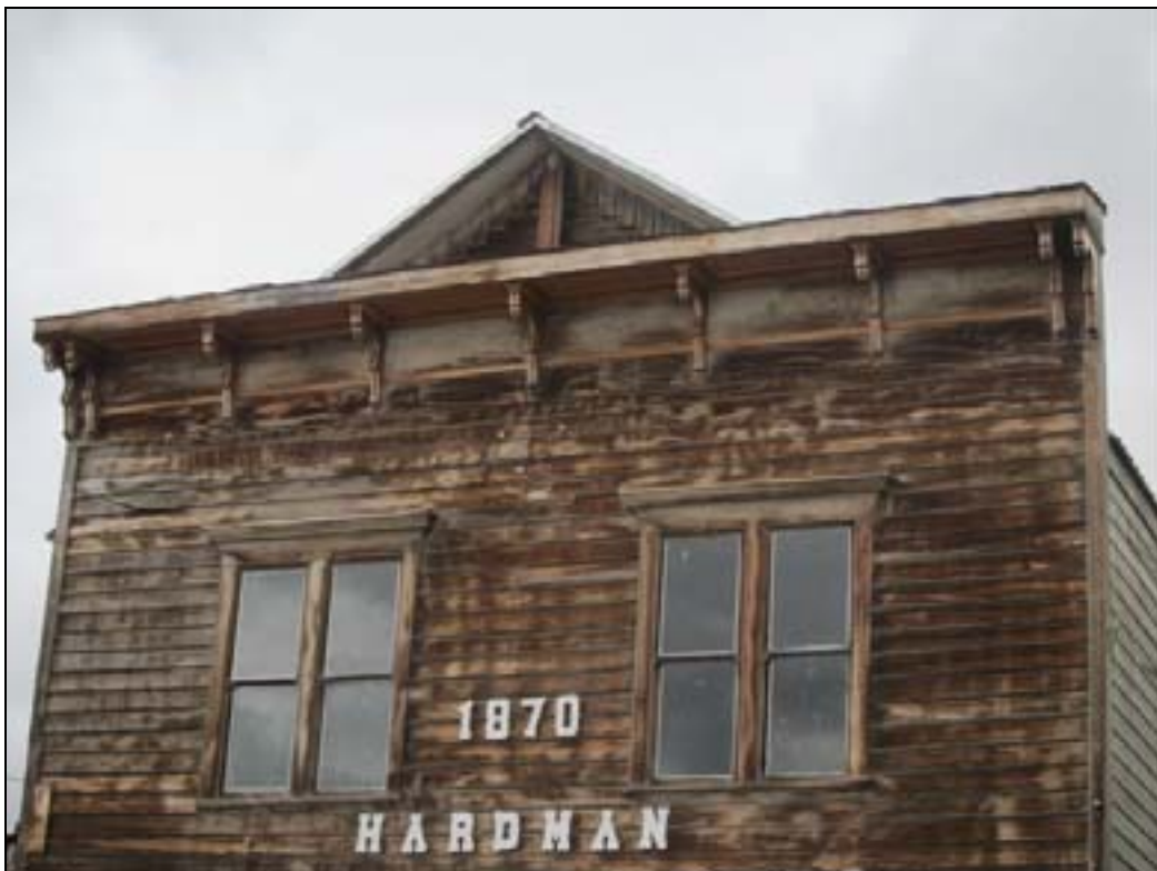
Photo 2 of 16: (OR_MorrowCounty_HardmanIOOFLodge_0002) East façade of the Hardman IOOF Lodge showing second story windows, cornice detail, decorative brackets, and gable end detail.
